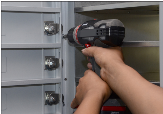
Figure 12 – 4C Connector Bar is now attached to mailbox unit
