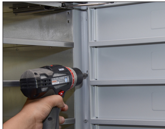
Figure 16– Secure units together using connector machine screws
