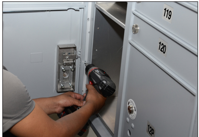
Figure 12 – 4C Connector Bar is now attached to mailbox unit
