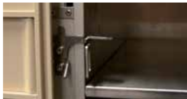
Easy release handle to open master gate
