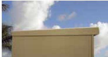
Sloped top for moisture runoff
