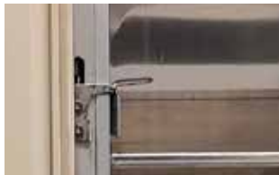
Easy release handle to open master gate
